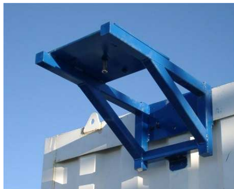
Figure 20 · The support on the side of the Meteorological Hut
